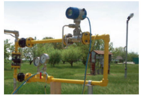
Mobile metering system with a flanged OPTISWIRL 4070 C
