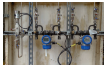
OPTIBAR DP 7060 (centre) as well as gauge pressure measurement with the OPTIBAR PM 3050 (left)
