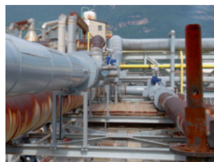
Start of the utilities towards the chemical plant
