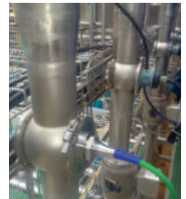
Inductive conductivity measurement of cleaning agents
