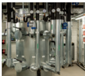
Concrete core temperature control
