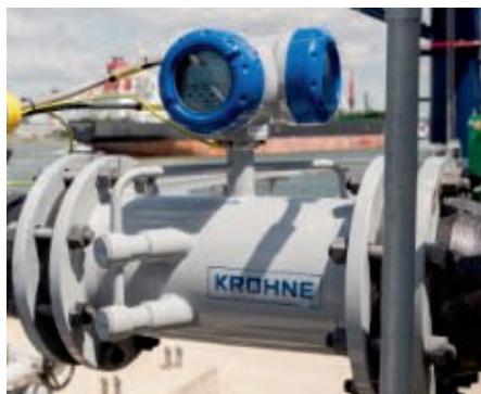
Ultrasonic flow measurement of hydrocarbon vapors
