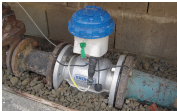
Measuring tube supported by gravel bed
