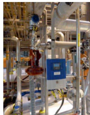
Electromagnetic flowmeters on water circuits
