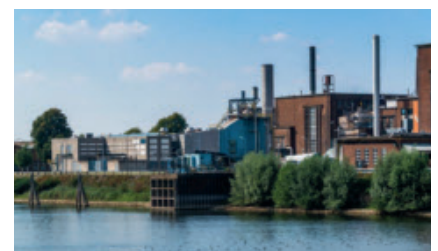
Historic boiler house with new biomass boiler in the Industrial Park Kleefse Waard (IPKW)
