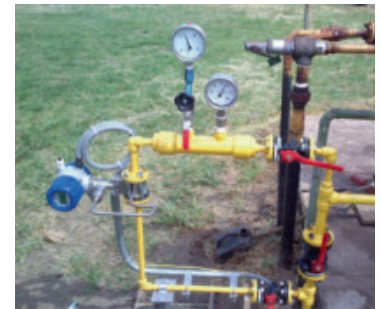
Installation of flowmeter with sandwich connection
