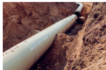
Construction of a pipeline
