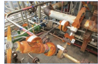
Retrofitted flange pressure tapping
