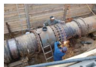
Welding work on the M960 from 1981
