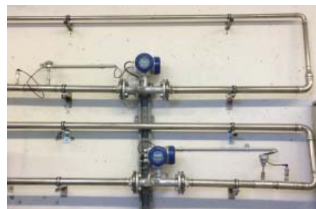
Ultrasonic flowmeters with pressure transmitters and temperature assemblies
