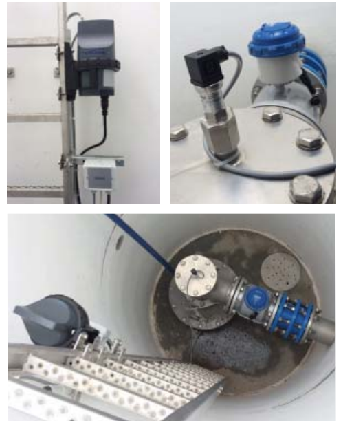
Top left: Data transmission with KGA 42; Top right: OPTIBAR P 1010 C and WATERFLUX 3070 C; Bottom: OPTIBAR LC 1010 C submersible level probe installed in a well shaft.
