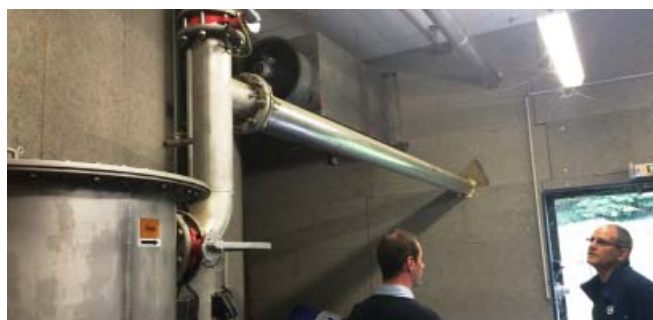
Inspecting the measuring point
