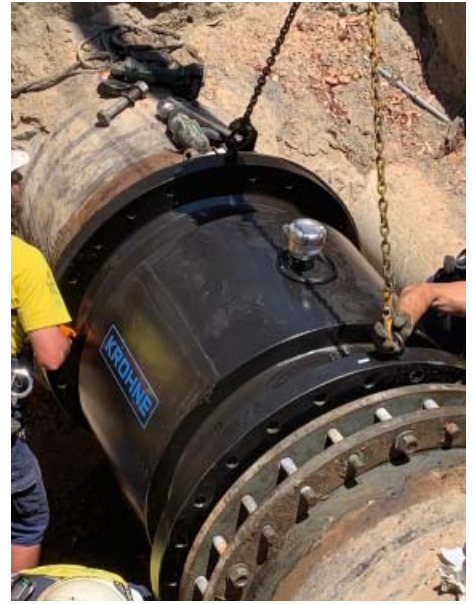
OPTIFLUX 2300 W with special burial coating
