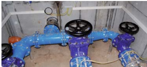
Splitting the main water line into 3 supply lines
