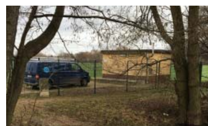
ZVO pumping station
