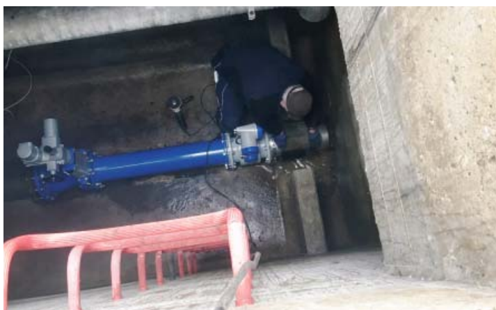
Installation of the measuring technology
