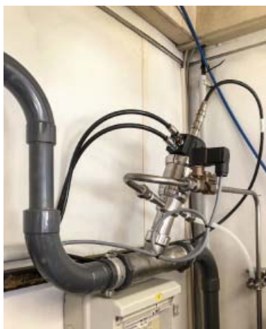
pH measurement with the SMARTPAT PH 8320
