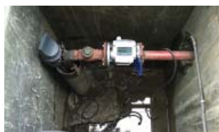
WATERFLUX 3070 C and KGA 42 installed at different sites
