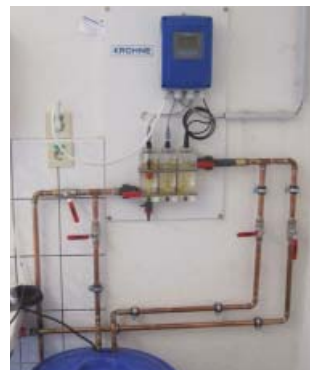
OPTISYS CL 1100 with measuring and flushing circuit
