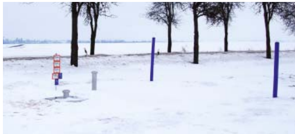
An extremely remote distribution shaft: there is no chance of supplying the measuring devices here with an external power supply
