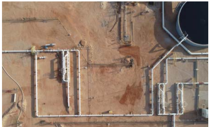
Metering system at the inlet of the water treatment plant
