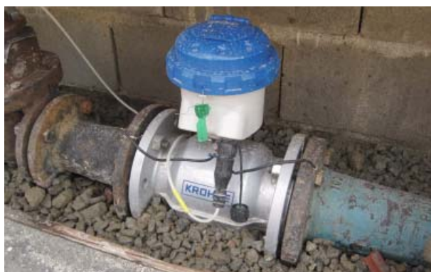
Measuring tube supported by gravel bed
