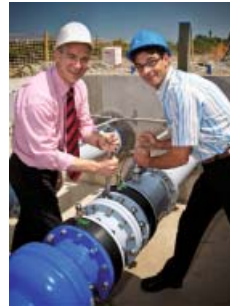
Final installation of the meter
