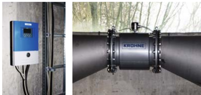
Wall version of converter (left) and sensor (right) of the WATERFLUX 3300 W electromagnetic flowmeter
