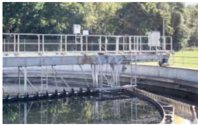
OPTISYS SLM 2100 and KRL 70 on the scraper bridge
