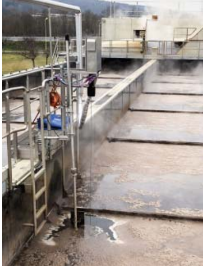
Measuring the sludge level in the clarifier
