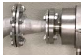
Installation in tapered pipe
