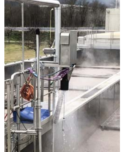
Integrated flush cleaning for the sensor
