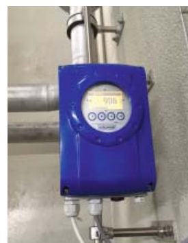
Flocculant measurement with the OPTIFLUX 1050
