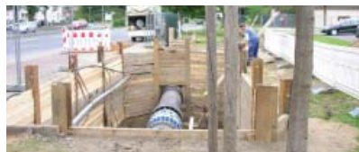
The flange-mounted OPTIFLUX 2300 with virtual reference
