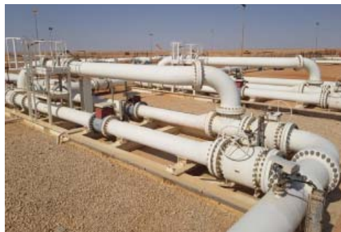
Metering system at the inlet of the water treatment plant
