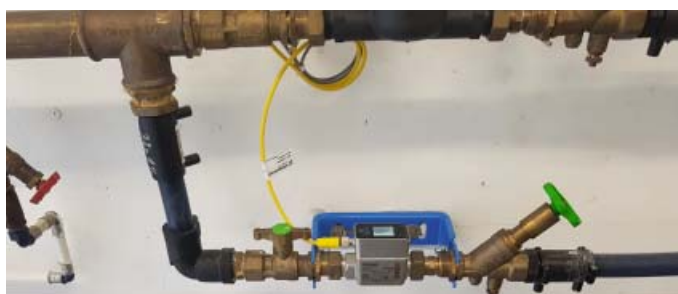
Electromagnetic flow measurement for optimising cleaning processes in preliminary treatment
