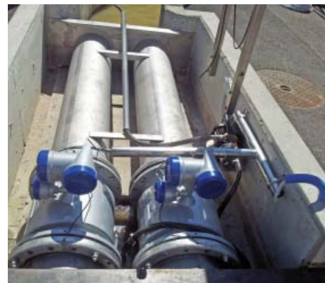
Installation of TIDALFLUX 2300 in sewage channel
