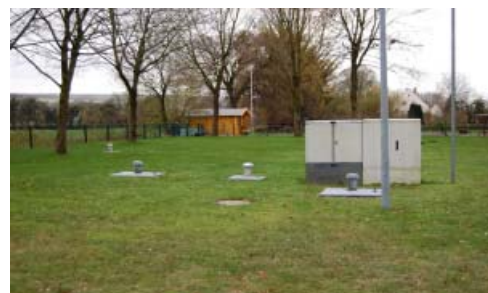
Ventilation shafts and control cabinets above the stormwater basin
