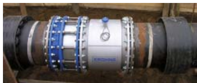
The flange-mounted OPTIFLUX 2300 with virtual reference
