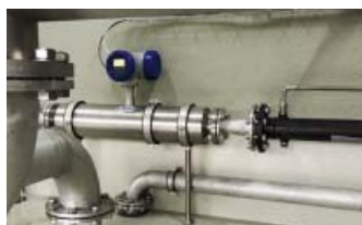
Measuring point with OPTIMASS 7400 C
