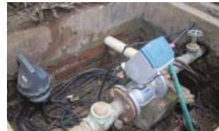
WATERFLUX 3070 C and KGA 42 installed at different sites
