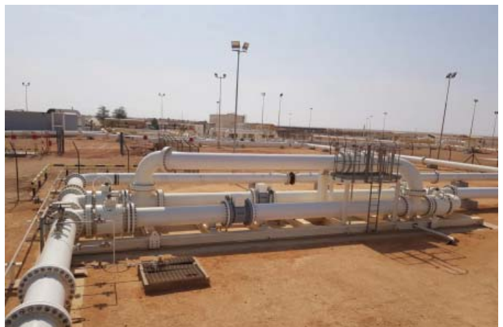
Water skids with the OPTIFLUX 2300
