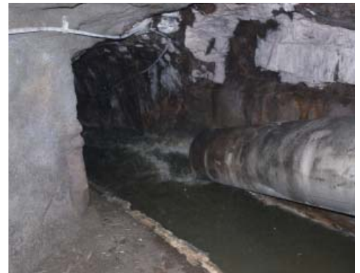
Outlet into wastewater tunnel system
