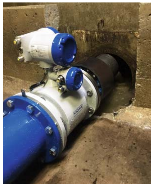
TIDALFLUX 2300 – Flowmeter for gravity pipelines
