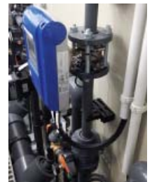
OPTIFLUX 5100 for dosing of sodium hypochlorite solution
