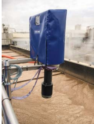
OPTISYS SLM 2100 with frost protection cover during winter operation
