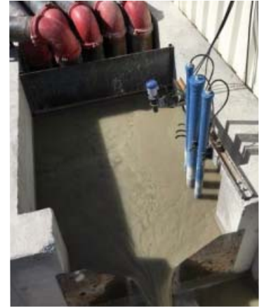
Measurement of pH, turbidity, conductivity and level
