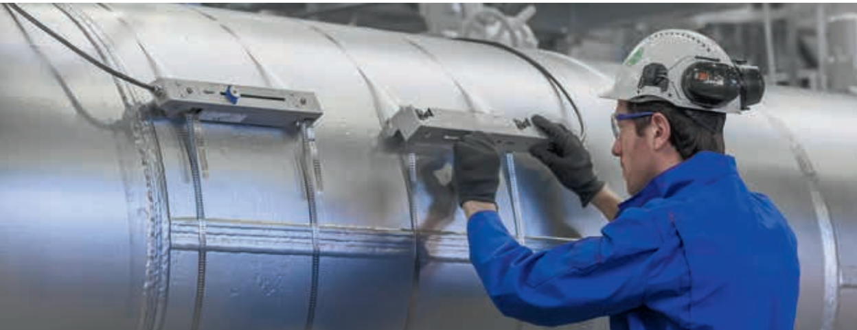
Clamp-on flow measurement on large line size
