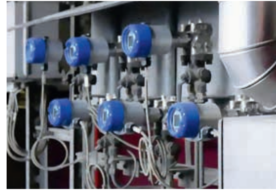
OPTIBAR DP 7060 differential pressure transmitters at a power plant
