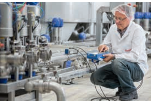
Temporary flow measurement with clamp-on flowmeter in a dairy
