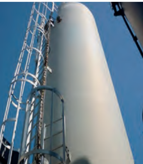
OPTIWAVE 6500 C with DN70; 2.75" PEEK Lens antenna and DN100 flange on the lime silo of a water treatment plant
