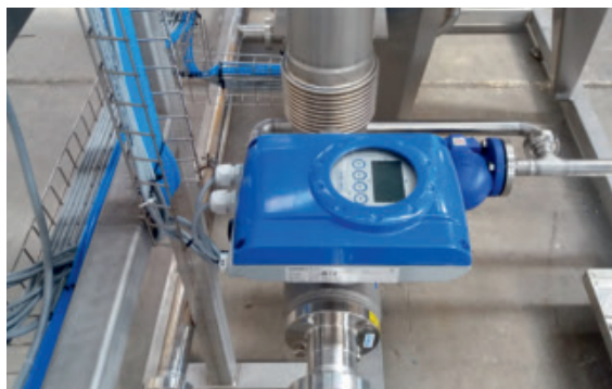
OPTIFLUX 6050 C on CIP skid unit
