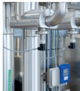
Conductivity measurement with the OPTISENS COND 1200 and MAC100 signal converter
