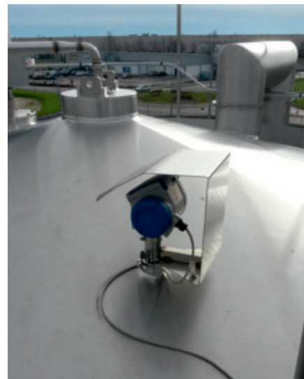
OPTIWAVE 7300 C with hygienic Tri-Clamp connection
