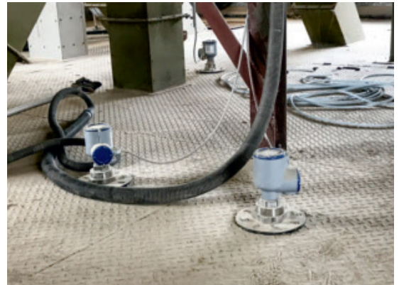
Level measurement in raw feed and grain silos
