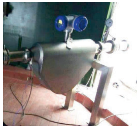
Installation of OPTIMASS 6400 (DN100 / 4") with SMS connections for hygienic flow measurement of bright beer
