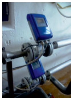
Water flow measurement with the WATERFLUX 3100 C
