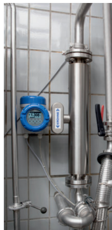
Brix measurement with the OPTIMASS 7300
