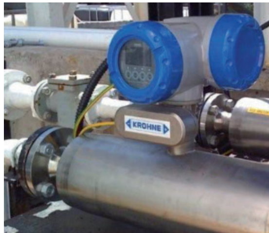
The OPTIMASS 7300 C with integrated concentration measurement
