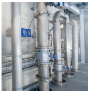
Flow measurement of dairy wastewater with the OPTIFLUX 2100 F
