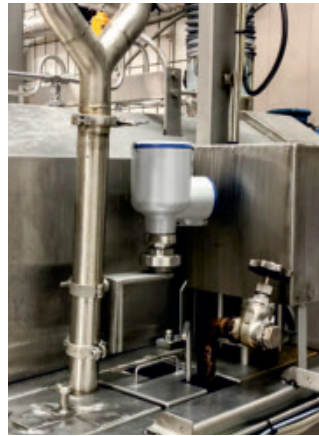
Level measurement of hot edible oil
