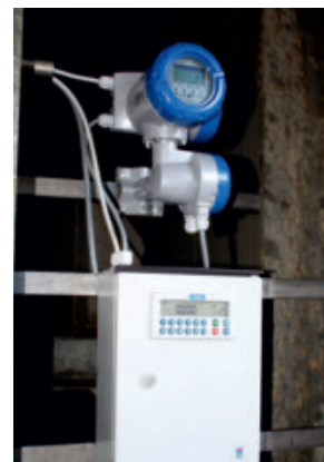
Converter (field housing) of OPTIMASS 1400 F above, preselection counter below
