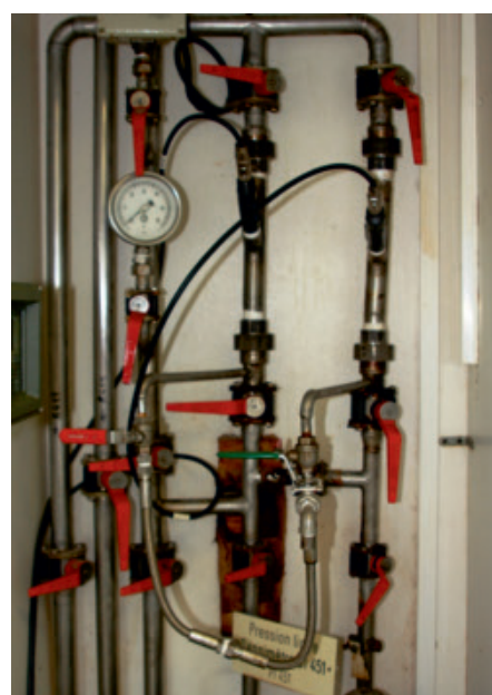
SMARTPAT PH 2390 installed between a hydrometer (left) and a redundant probe (right)
