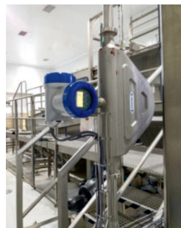
Flow measurement of tomato paste with the OPTIMASS 6400 C
