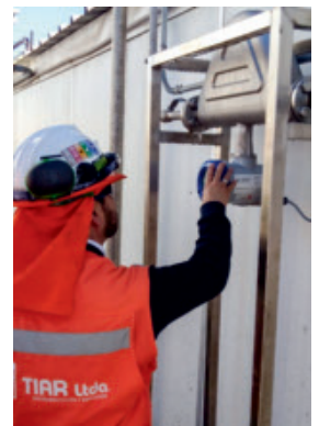
Installation of the flowmeter
