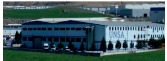
Ünsa Makina manufacturing plant
