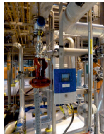
Electromagnetic flowmeters on water circuits
