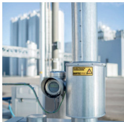
Flow measurement at the raw milk reception with the OPTIFLUX 6300
