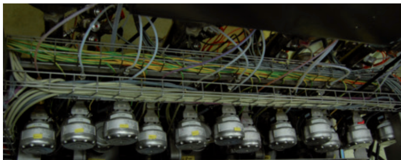
Measurement of the metered flavours using OPTIFLUX 6000 and OPTIMASS 3000.
