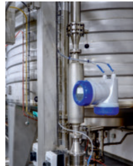
Picture above and right: OPTIMASS 7400 C with heating jacket; Picture left: OPTIMASS 1400 C
