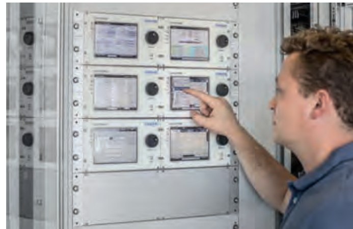
Supervisory control cabinets based on the SUMMIT 8800 flow computer
