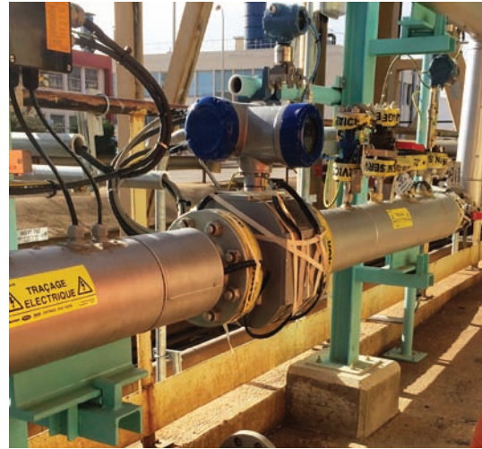
Custody transfer flow measurement with the ALTOSONIC V12 ultrasonic gas flowmeter
