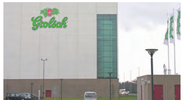
New construction of GROLSCH brewery near Enschede, the Netherlands
