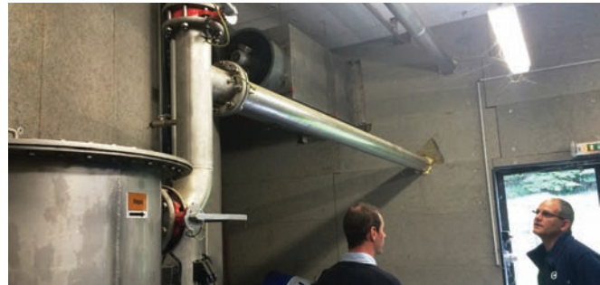
Inspecting the measuring point
