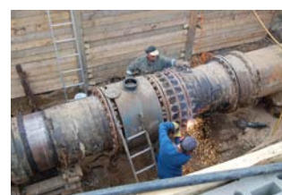
Welding work on the M960 from 1981
