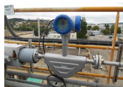
Measuring gas mixture with the OPTIMASS 6400 C
