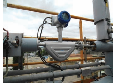
OPTIMASS 6400 installation
