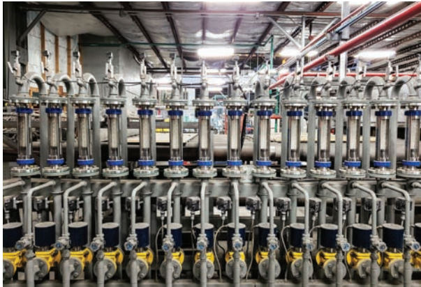
Hydrogen flow measurement with the VA 40 variable area flowmeter
