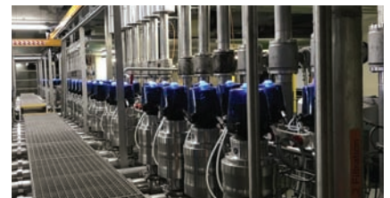
Monitoring the filling and emptying of beer tanks
